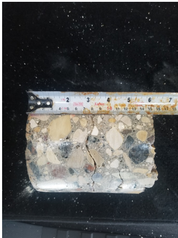
Photograph 12: Test Hole TH19-25 - McDowell Drive
