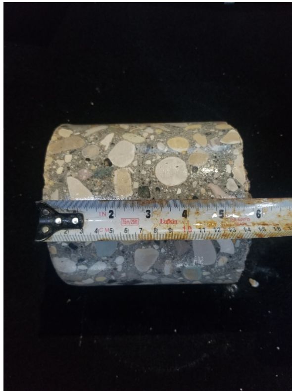
Photograph 8: Test Hole TH19-21 - McDowell Drive
