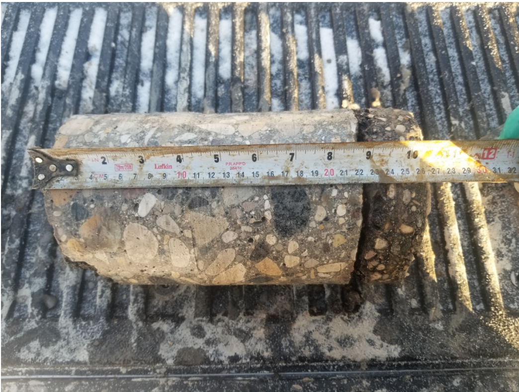
Photograph 4: Test Hole TH19-17 - Lanark Street
