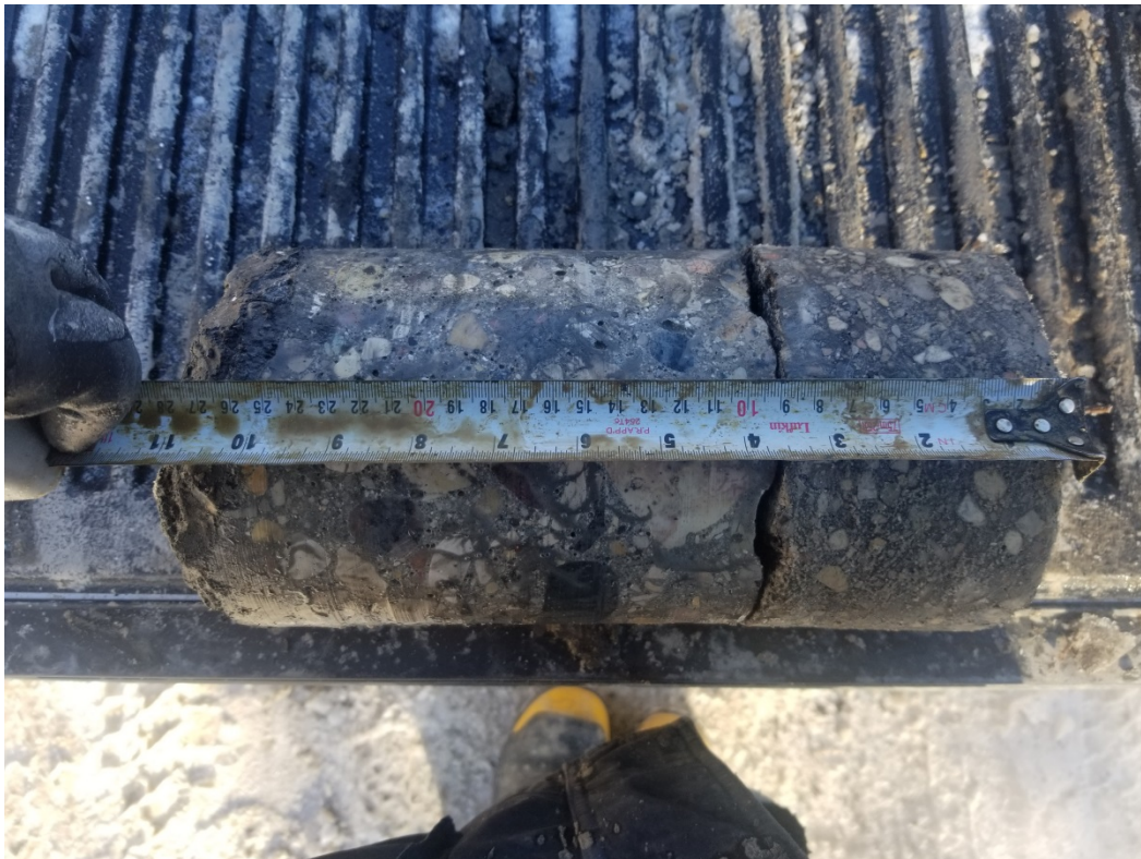
Photograph 2: Test Hole TH19-15 - Lanark Street
