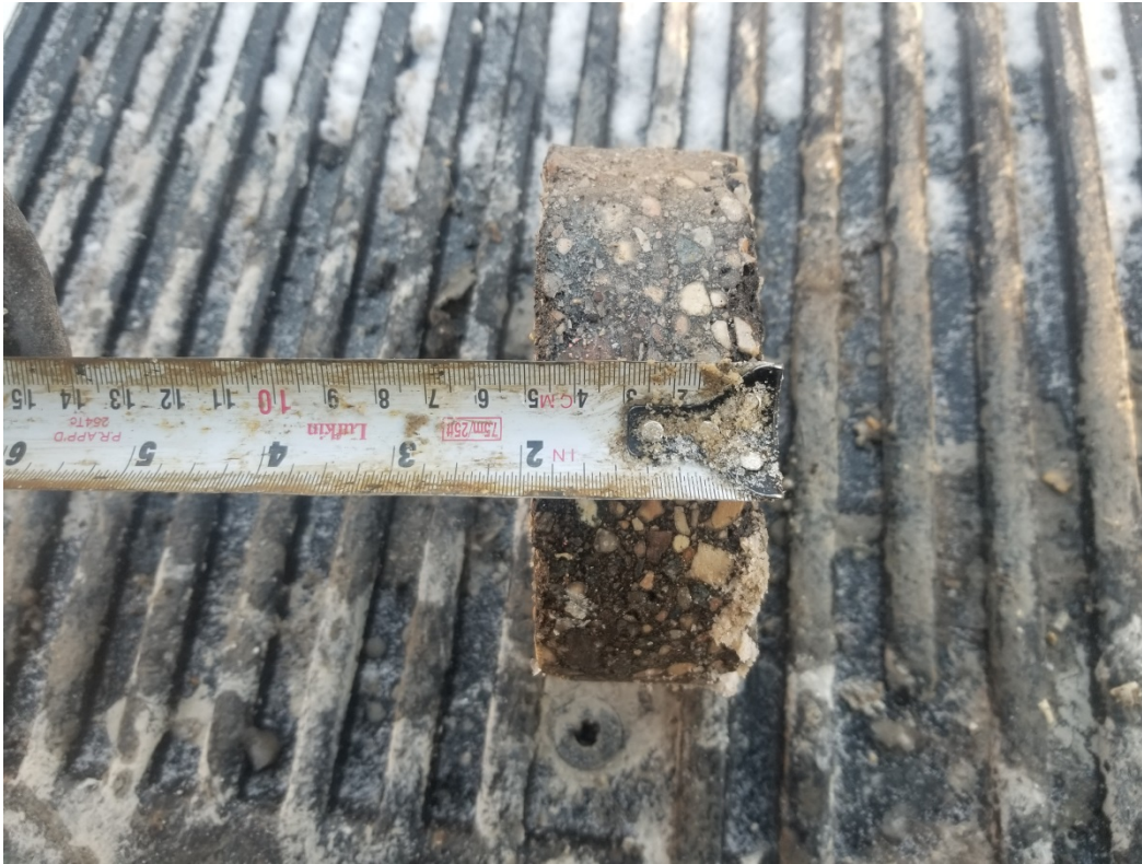
Photograph 3: Test Hole TH19-16 - Lanark Street - Concrete not recovered
