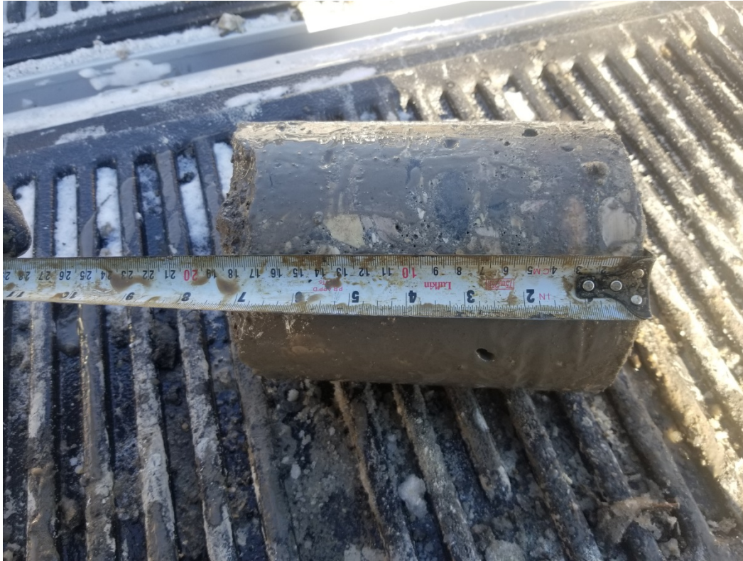
Photograph 1: Test Hole TH19-14 - Lanark Street - Asphalt not recovered
