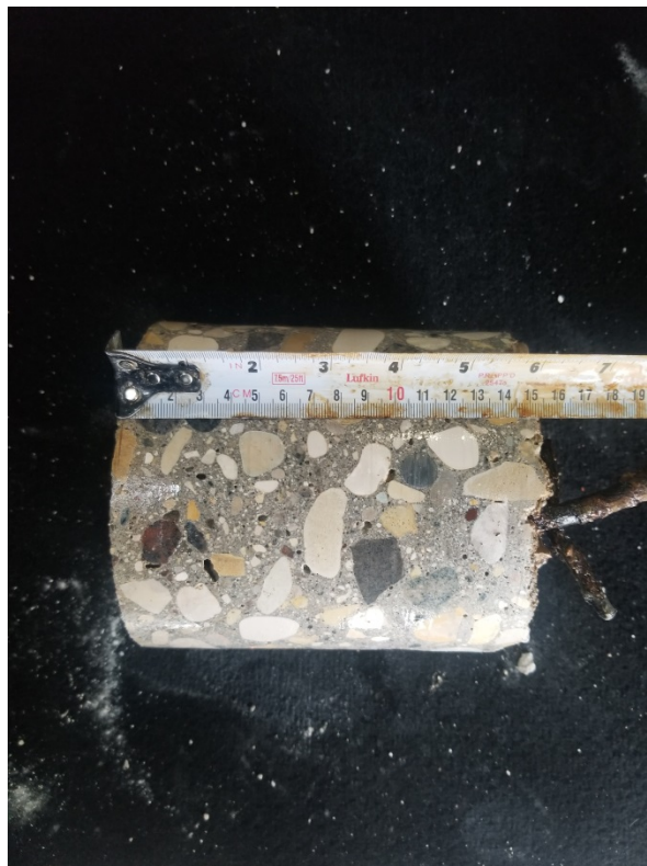
Photograph 10: Test Hole TH19-23 - McDowell Drive
