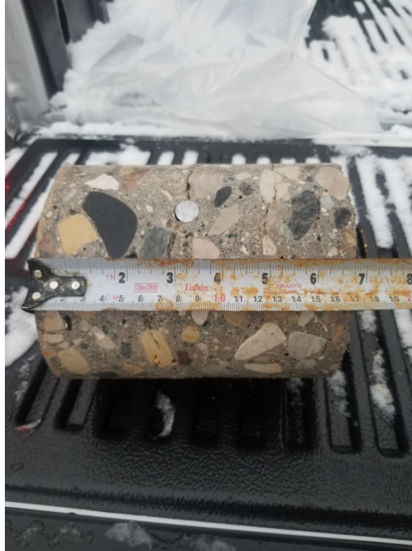
Photograph 7: Test Hole TH19-20 - McDowell Drive
