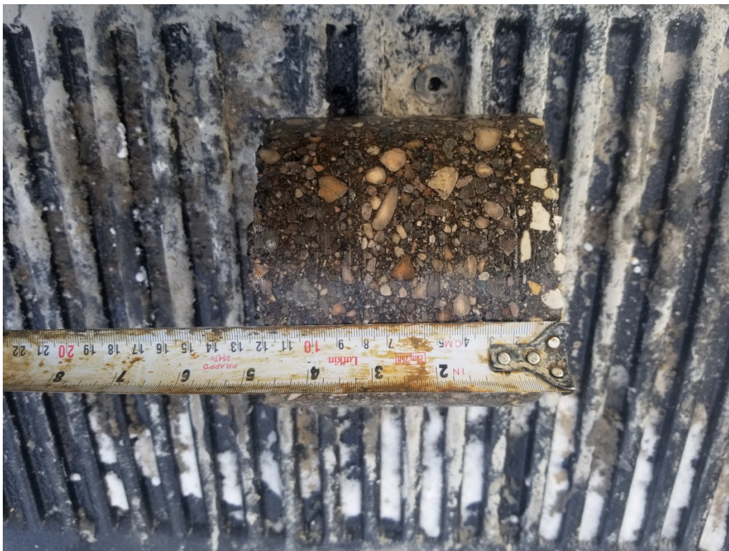
Photograph 14: Test Hole CH19-34 - Mountbatten Avenue - Concrete not recovered
